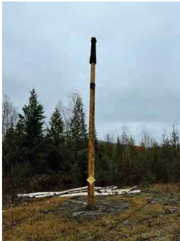
12 - Finished installation of BrandenBark on a pole. Photo: H. Gates.
