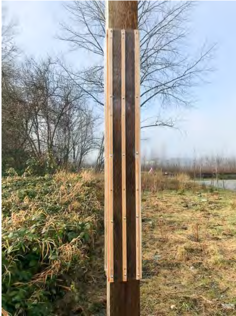
18 - Photo 6: Predator guard strips mounted on narrow wood material (Blakeburn)
