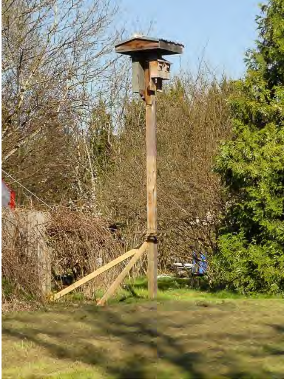
19 - Photo 7: Braces attached to bat post (Pitt Meadows)
